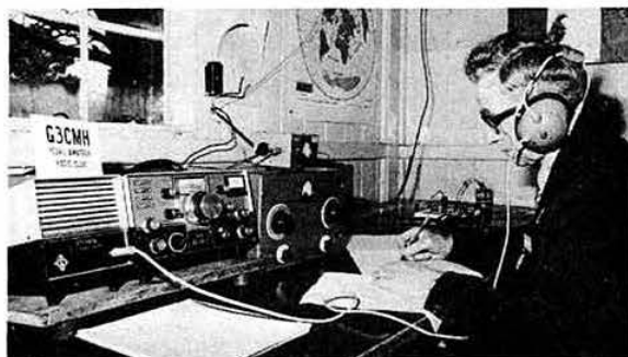
G3BCC operating the Yeovil Amateur Radio Club station G3CMH to commemorate the 25th anniversary, on 21 February, of the first long-distance short-wave contact in Britain using a transistor transmitter. The QRP transmitter is on the right, and the best distance worked with 38mW was G3EUE at 116 miles. The QRP station is operational on 3-549MHz on Thursdays at 1945bst.
